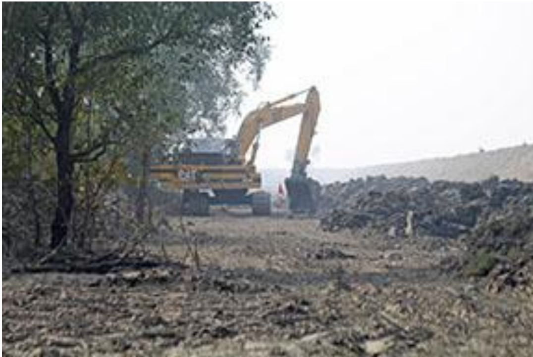
Construction of road in coastal mangroves.
