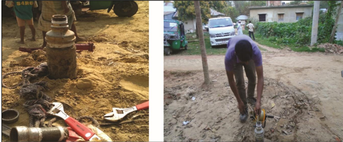
Figure 4: Established Monitoring well with 3 Inches Housing Pipe.
