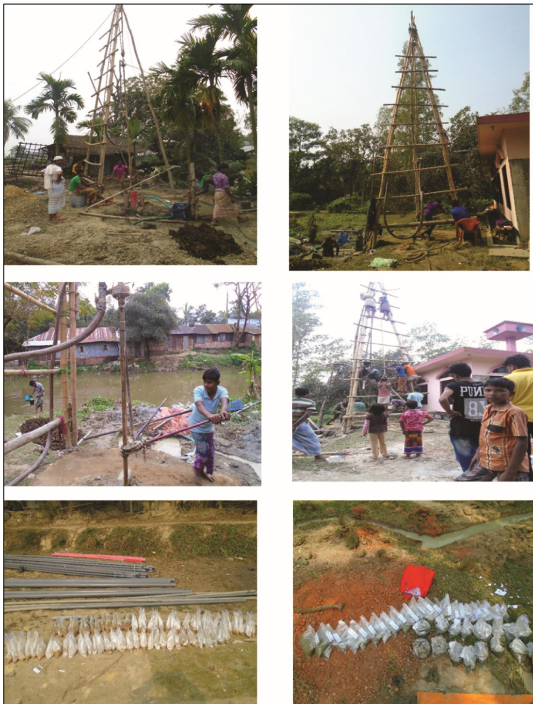
Figure 3: Monitoring well drilling and Wash samples.
