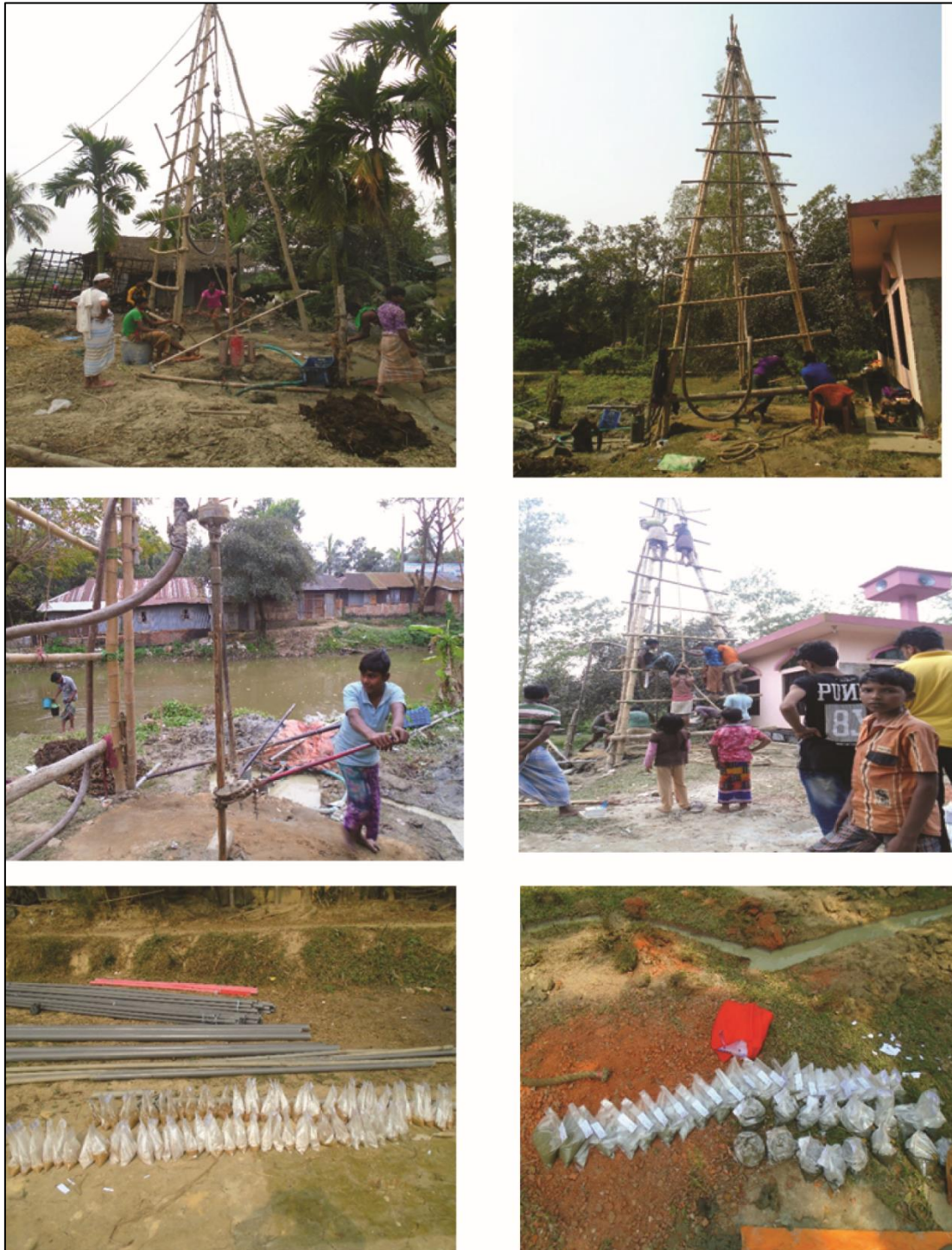
Figure 3: Monitoring well drilling and Wash samples.
