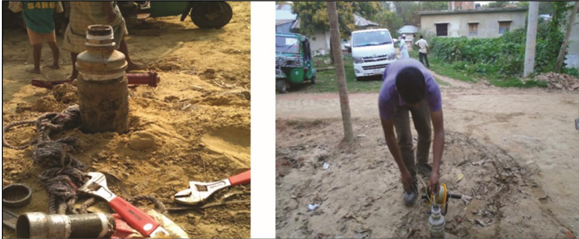
Figure 4: Established Monitoring well with 3 Inches Housing Pipe.
