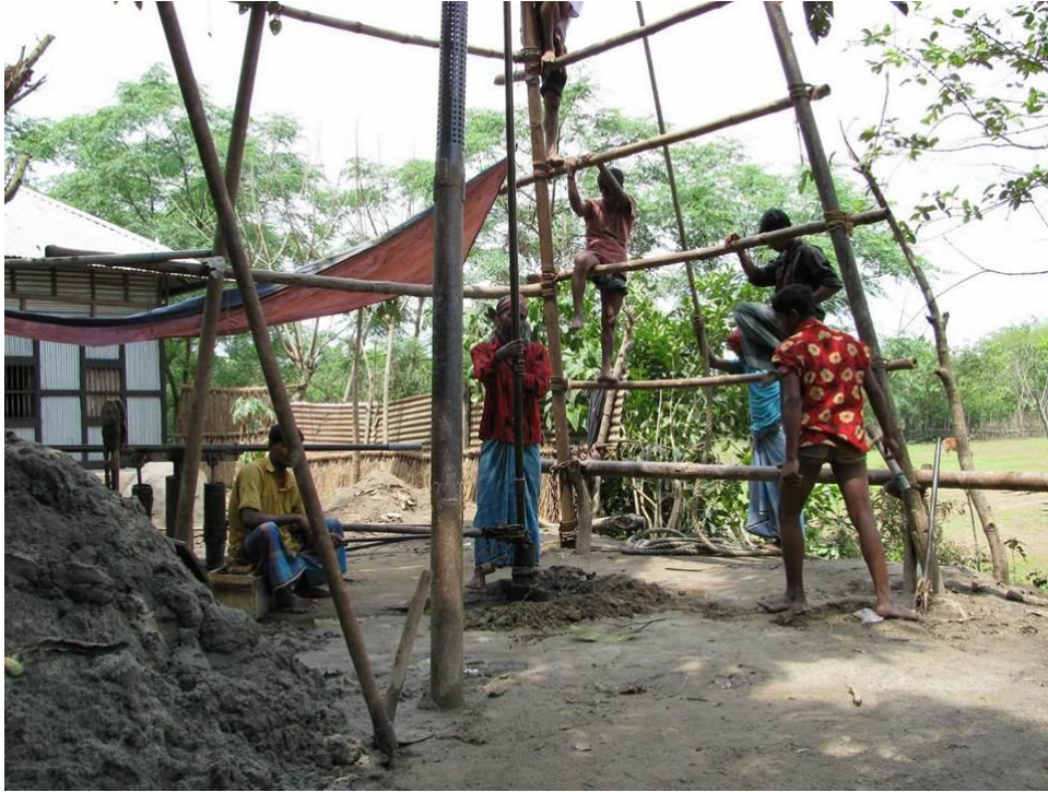
Figure-5: Drilling setup reverse circulation method.
