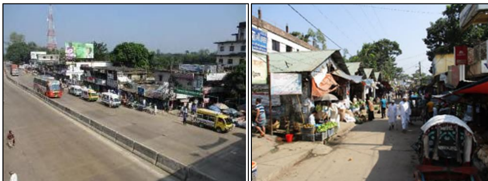
Photograph 3.4: Mirsharai Intersection and Zila Road towards Fatikchhari from the Mirsharai Intersection
