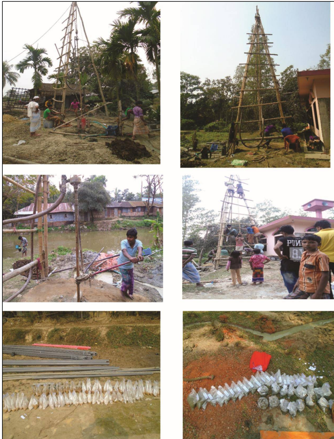
Figure 3: Monitoring well drilling and Wash samples.
