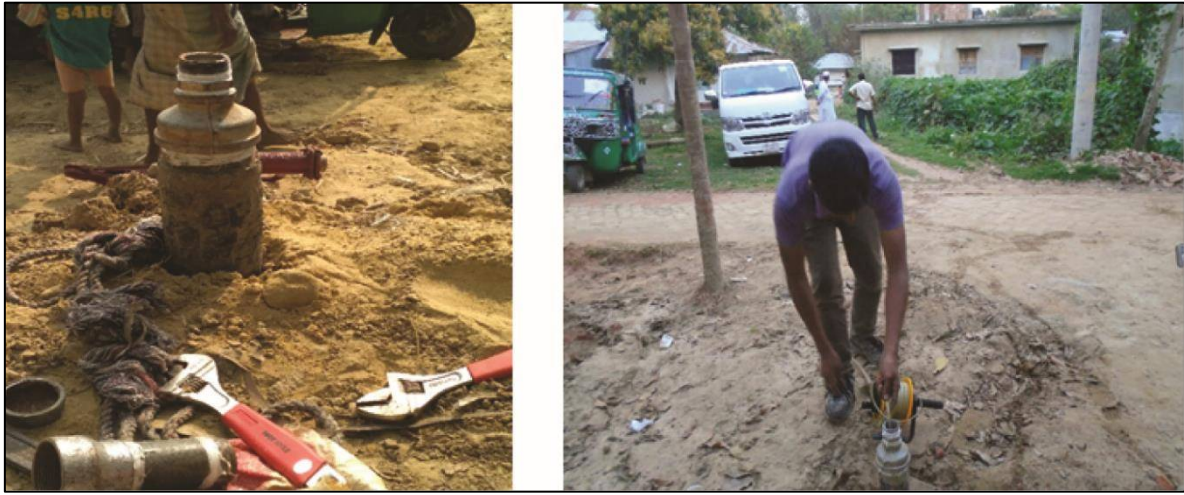
Figure 4: Established Monitoring well with 3 Inches Housing Pipe.
