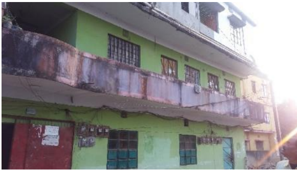
Camera location for VC at Mirsharai Paurashava (Upazila Road)
