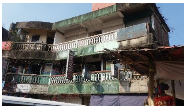
Camera location for VC at Baraiyarhat Rail Crossing
