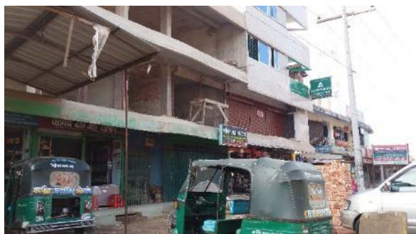
Camera location for VC at Muhuri Project Road
