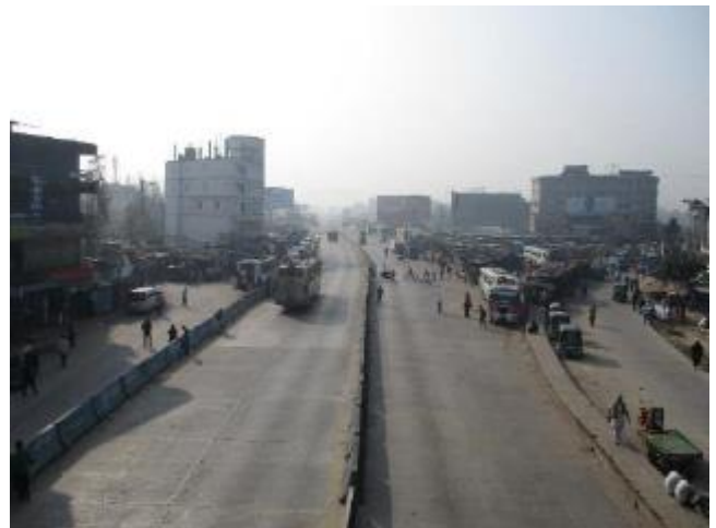
Baraiyar hat intersection (N1), one of the busiest
