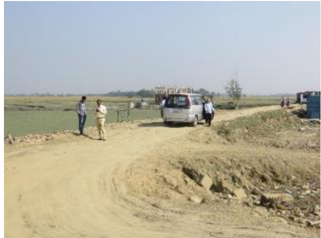
New Embankment Road within the EZ site
