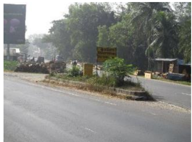
Mithachara intersection on Dhaka-Chittagong highway
