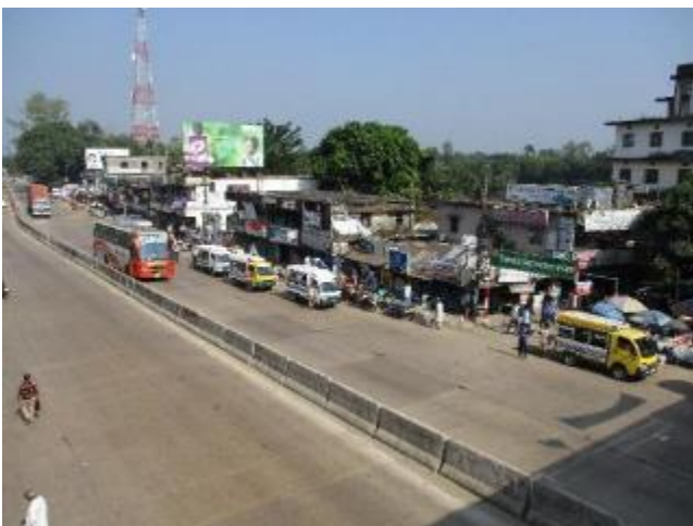
Mirsharai intersection on the highway
