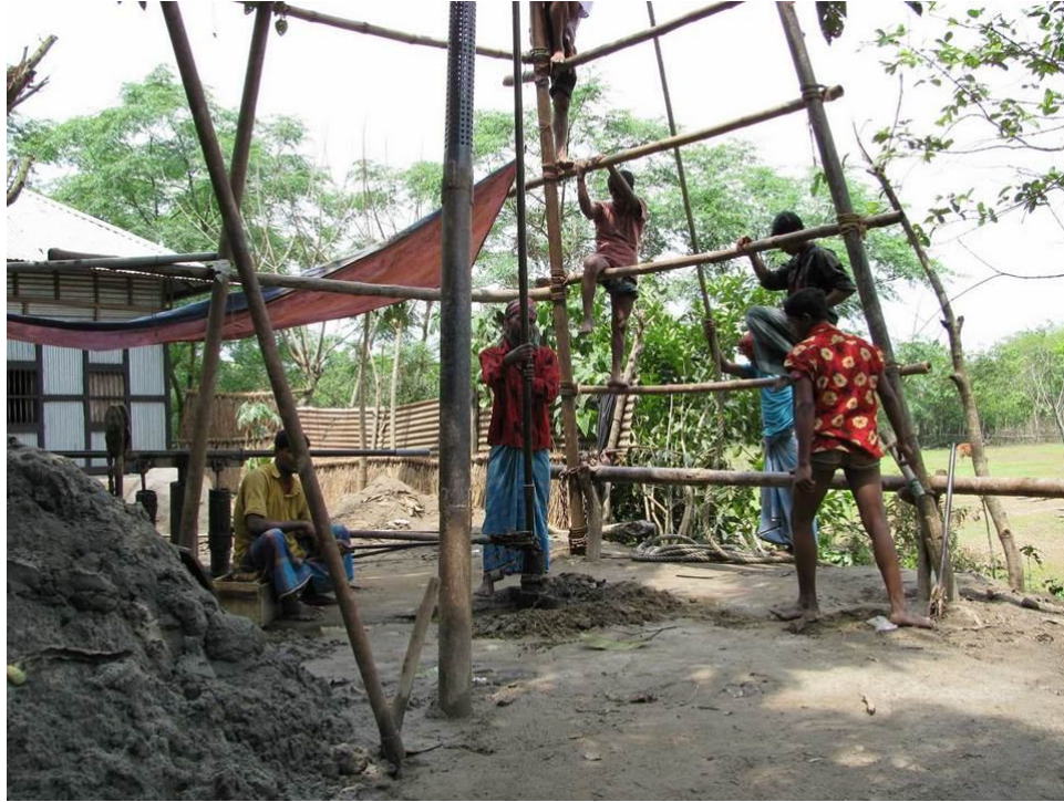
Figure-5: Drilling setup reverse circulation method.
