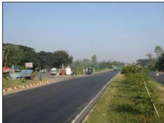
Photograph 3. 2: Chaitanner Hat Intersection
